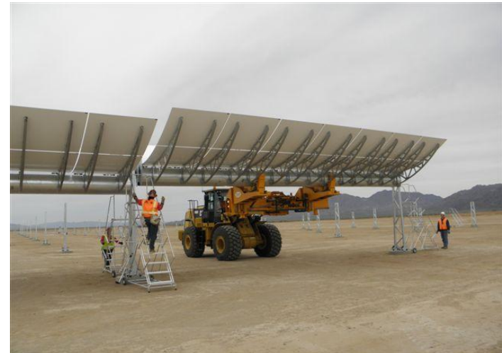
Solar Collection Element Installation
