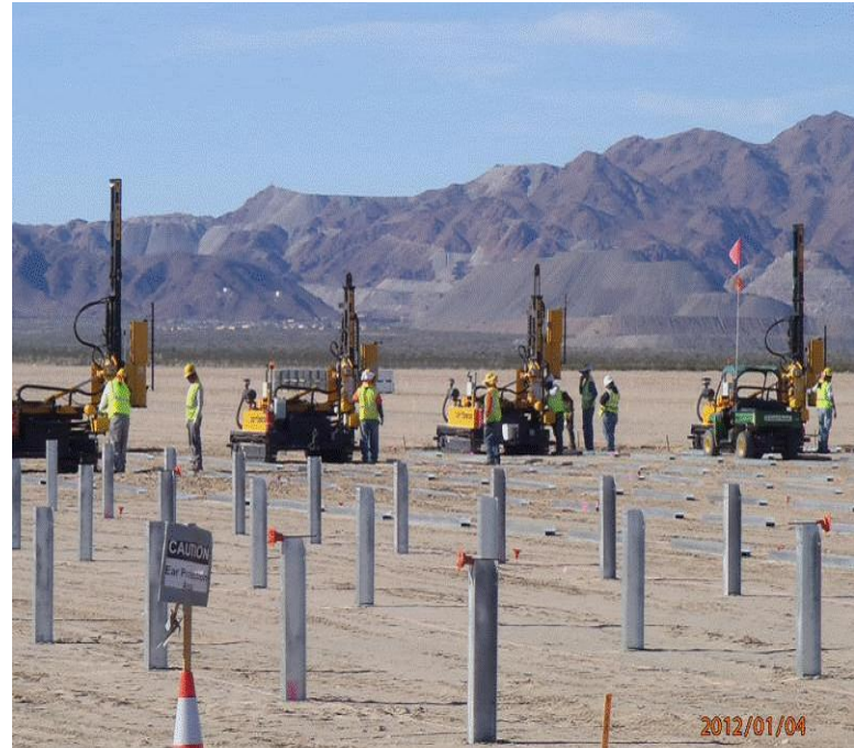
Post preparation and installation
